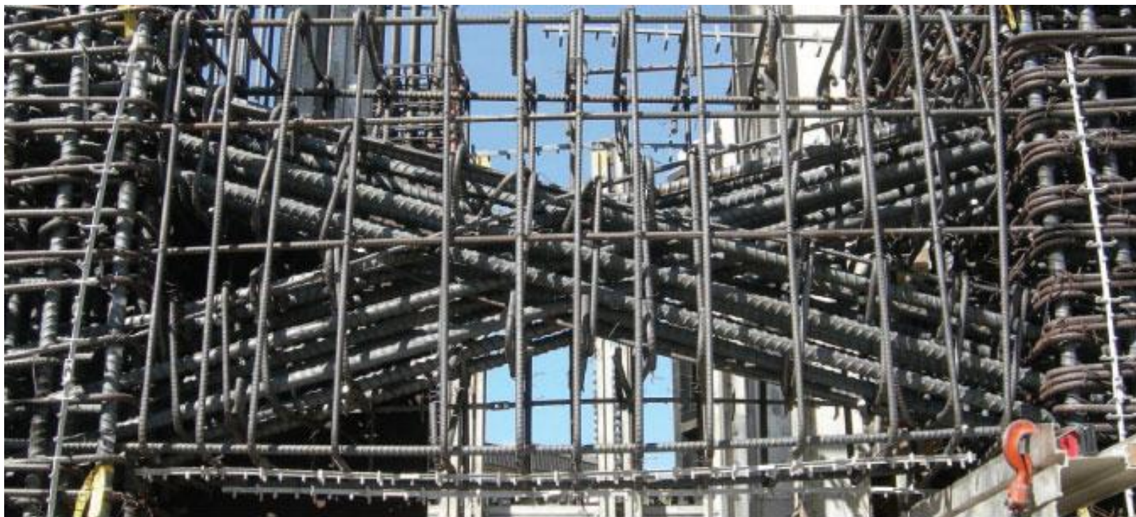
▲ Figure 1 Showing the intricate, labor-intensive steel reinforcing bar congestion in a typical high-rise coupling beam. Photo credit: Remy Lequesne, The University of Michigan
