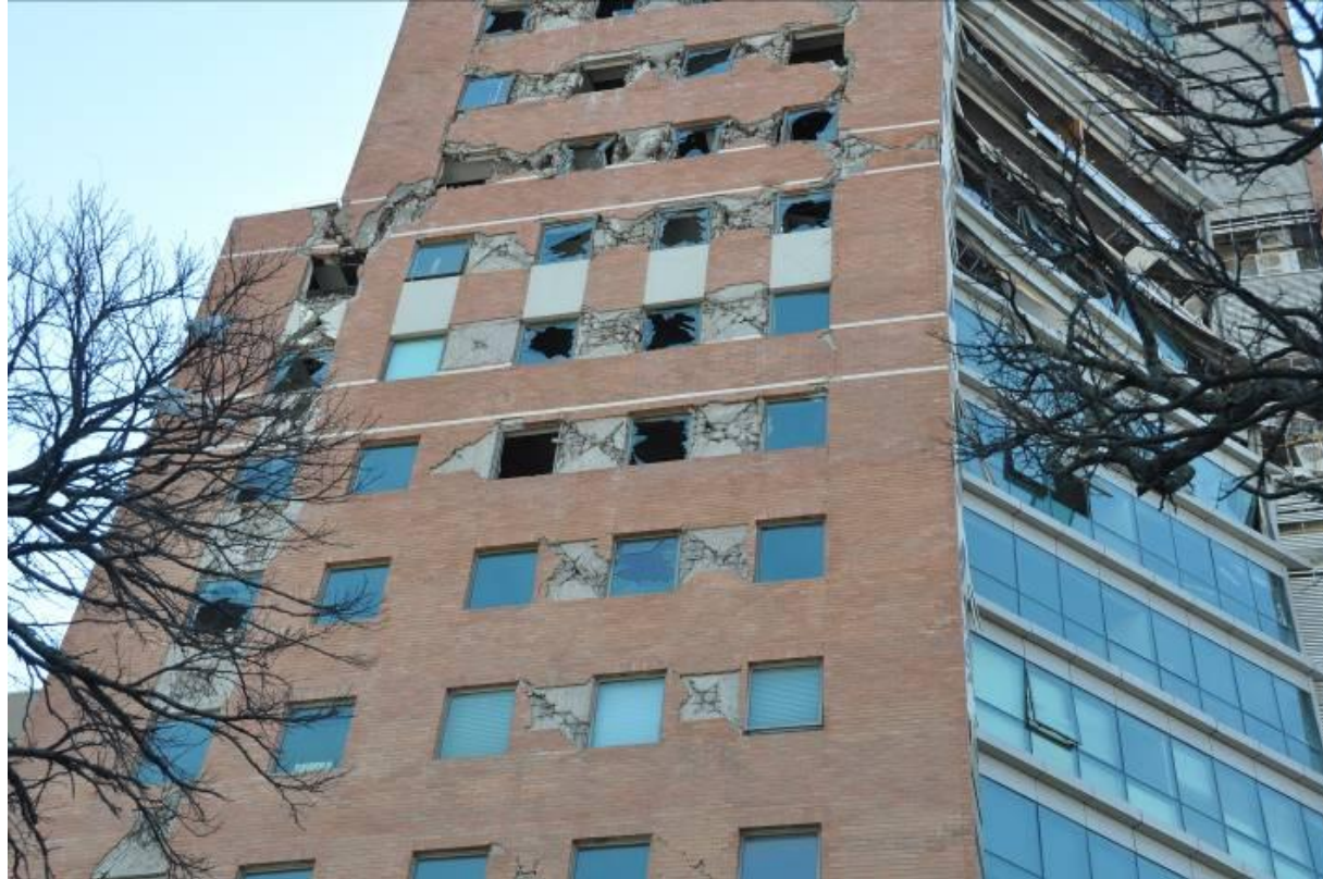
Torre O'Higgins Building Damaged by 2010 Chile Earthquake
